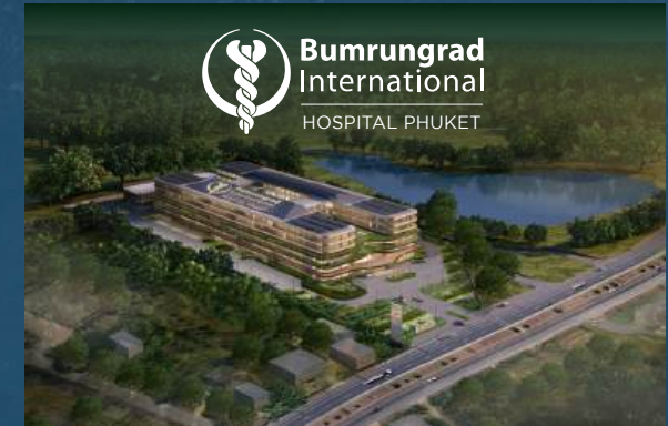
Bumrungrad International Hospital Phuket (under construction) 10min
